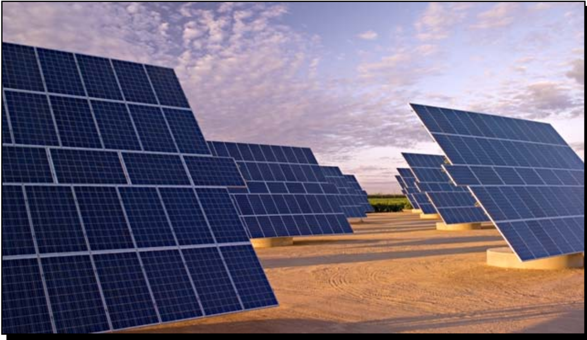
City of Madera Wastewater Treatment Facility, 1.16MW Dual Axis Trackers, California
